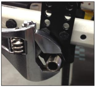
**Step 3:** Using a 1/2" socket and a 1/2" wrench, remove the OEM 5/16" bolts from the axle bracket.
